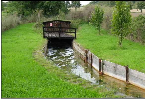
Abb. 3.3.2.3.-4: Mundloch des Schlüssel-Stollens
