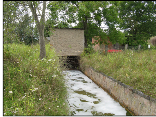
Abb. 3.3.2.3.-5: Mundloch des Schlüssel-Stollens
